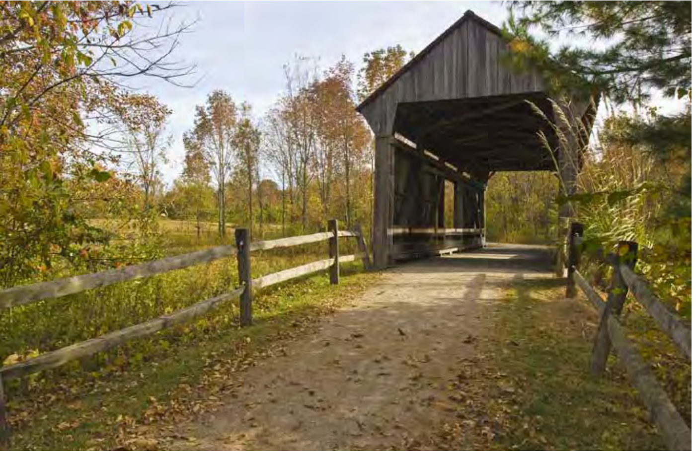
Covered bridge at Slate Run Metro Park
