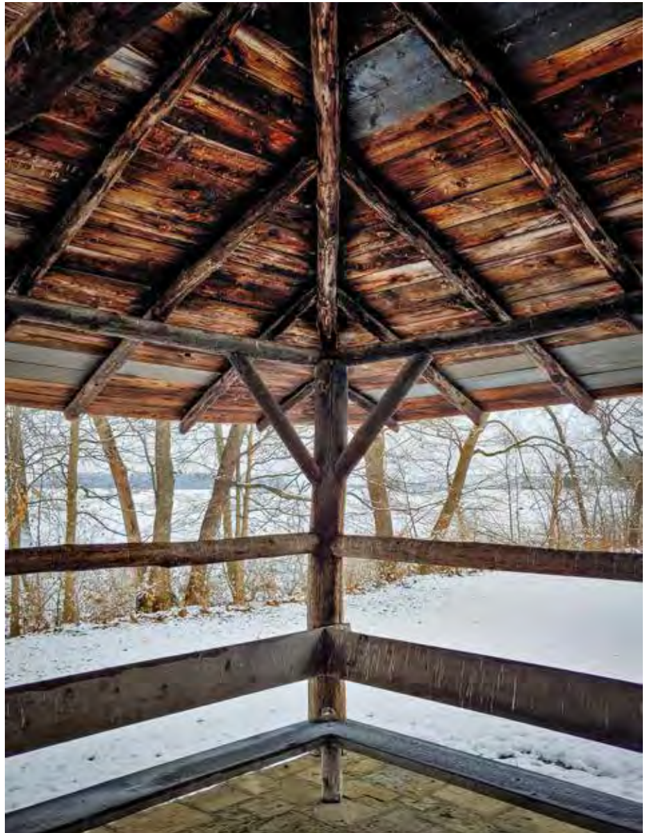
Shelter house at Logan Elm Park
