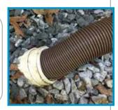
There are many ways to hook-up your sewer, but we recommend placing the sewer hose approximately 2 inches into the open sewer fitting.
